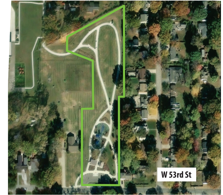
Figure 32: Located a few blocks west of Roeland Park on 53rd St in Mission, Water Works Park is a park developed under a joint-use agreement. Here, Water District #1 owns the land, and the City of Mission is responsible for its development and management as a public park. The park was established in 1982, and recently received a $2.4 million upgrade with new universally accessible play equipment, restrooms, lighting, landscaping, parking, and 10' wide fully accessible paths. Image Source, ESRI
