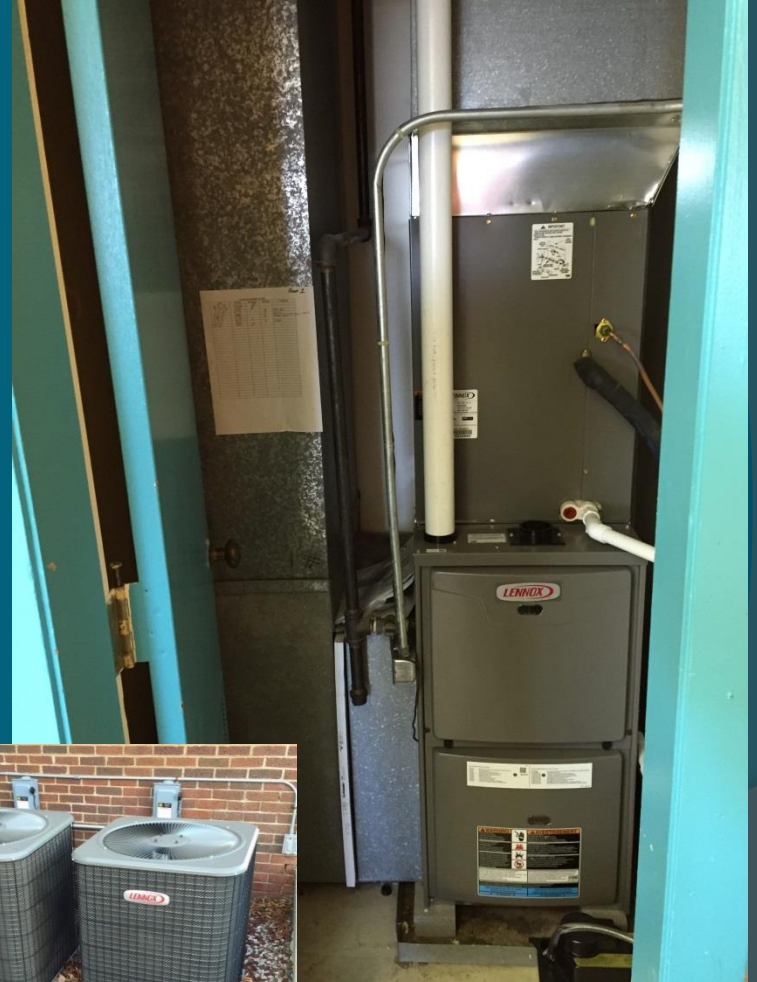
New condensing units installed for the MPR. New The Neighbors Place and Room 1.
