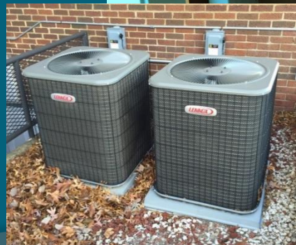
New condensing units installed for the MPR. New The Neighbors Place and Room 1.
