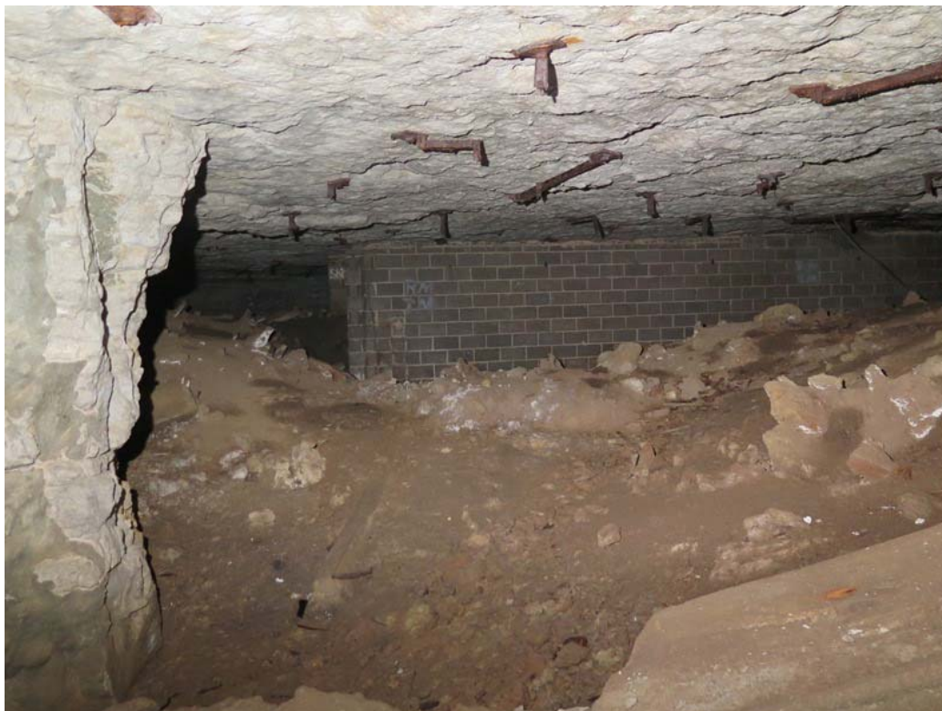
Photo 22: Looking west from inside Portal 2 towards masonry wall inside Portal 1. Pillar 4 shown on left. Old rockbolts and strapping visible in roof.
