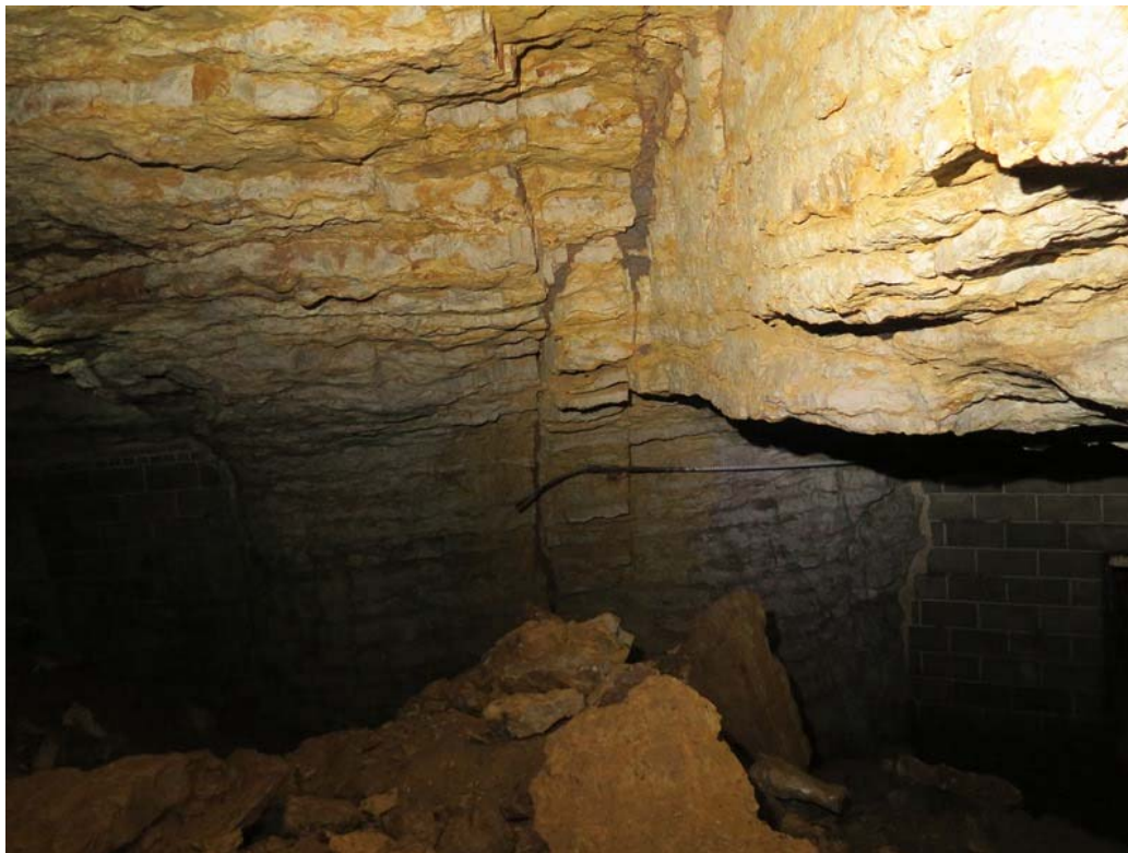
Photo 46: Looking west-southwest at parallel mud seams in the roof and Pillar 6.
