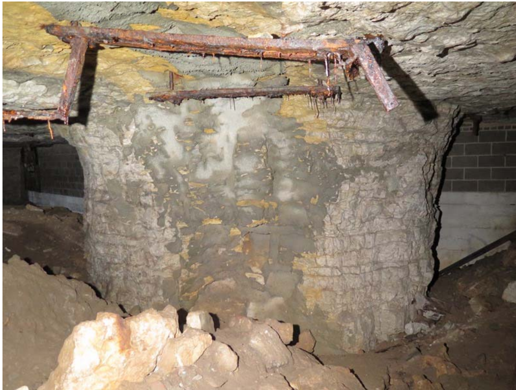
Photo 39: Looking northeast at Pillar 6. Gunite covers mud seam on roof and pillar. Masonry wall on left and right demarcates the boundary between the historically supported, recreational area on the west and the unsupported area to the east.
