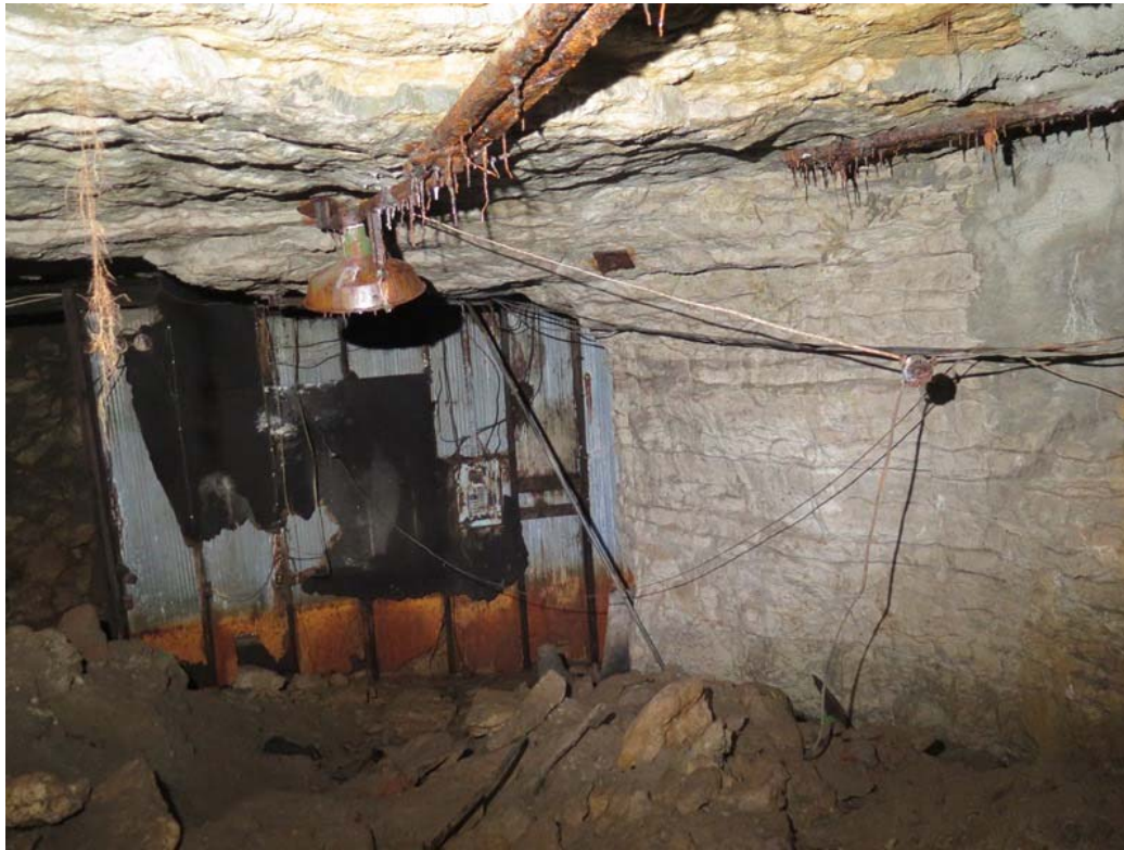
Photo 35: Looking south at wood framed, corrugated metal entry closure in Portal 3, Pillar 5 on right.
