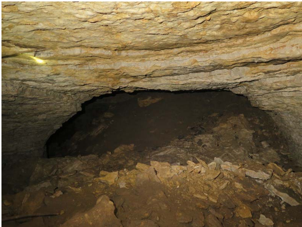
Photo 44: Looking east, Pillar 7 on left and Pillar 10 on right. Material in background is inside Portal 5.
