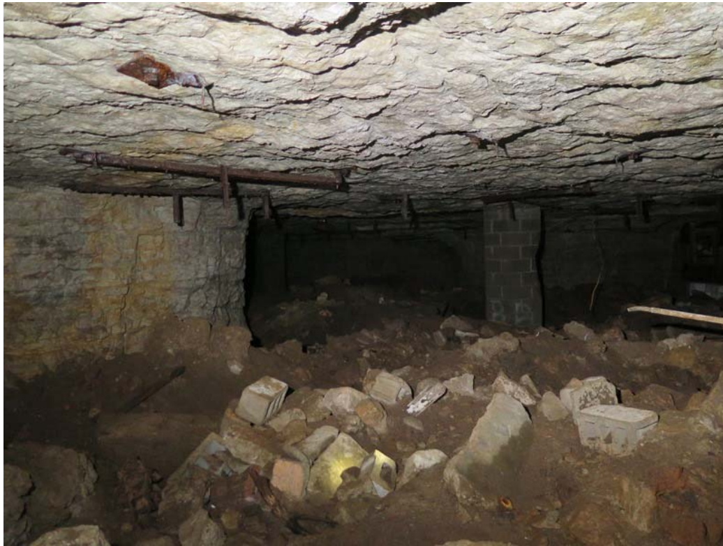
Photo 33: North (back) room inside Portal 3, Pillar 2 on left.
