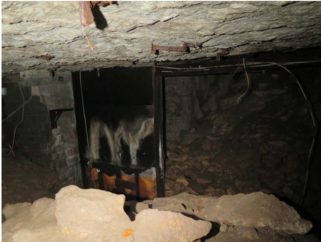
Photo 37: Looking southeast at remainder of corrugated metal closure in Portal 3 and Portal 3 backfill. Pillar 9 is shown near the center of the photo.
