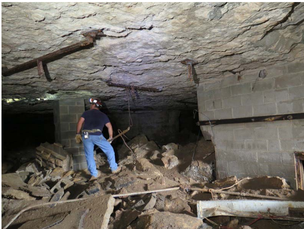
Photo 24: Looking northeast inside Portal 2. Pillar 3 is in center background, Pillar 5 is behind masonry wall on right.
