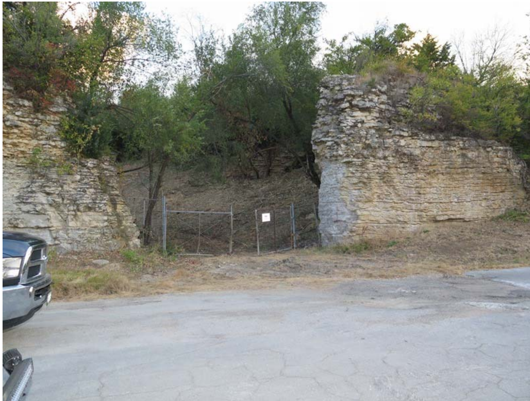
Photo 1: View between Pillars 13 & 14.
