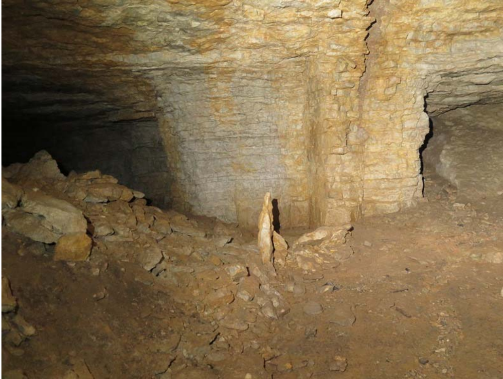
Photo 53: Looking east at mud seams in roof and Pillar 16 north of dome in Portal 5. Vertical rock slab in center of photo toppled from edge of the dome.
