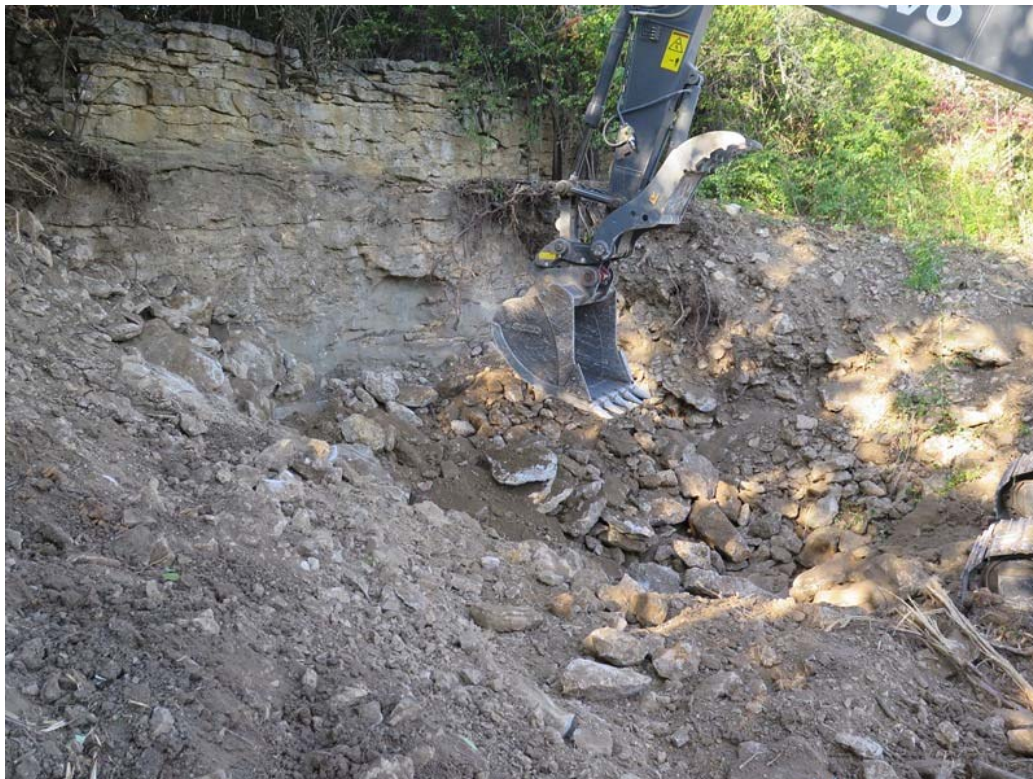
Photo 16: Portal 2 excavation secured at end of day, 10/20/15.
