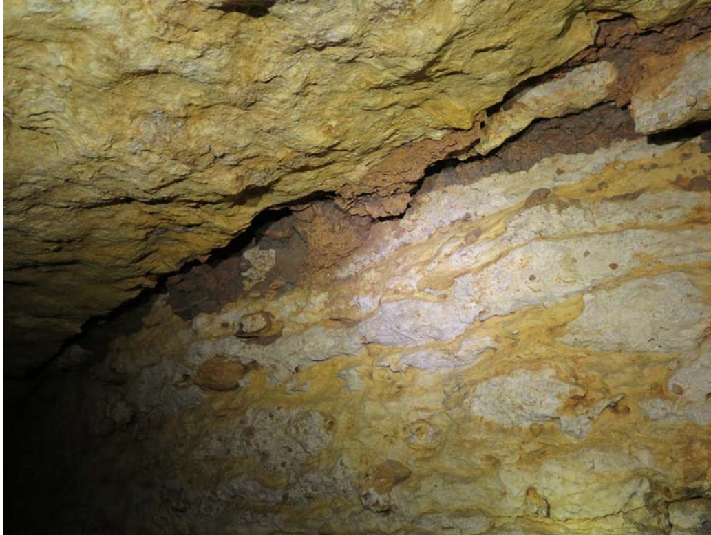
Photo 47: Looking northwest along the same mud seam (up to 8 inches thick) in the roof. The seam forms the north end of the Portal 4 dome.
