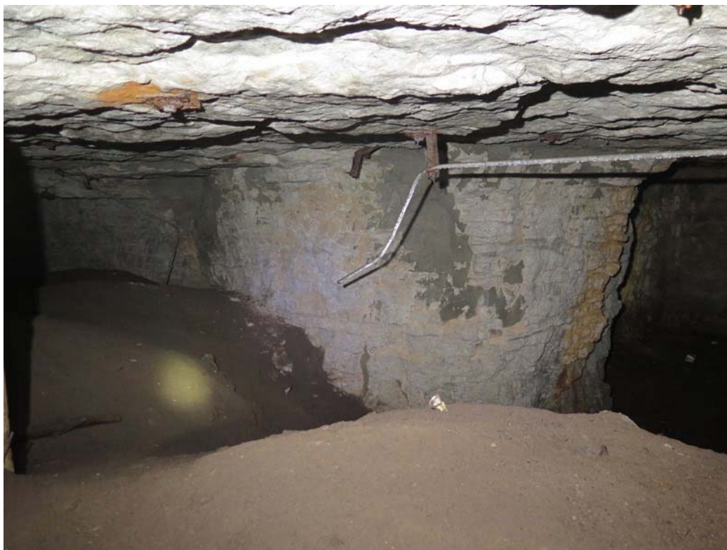
Photo 30: Looking northwest at Pillar 15.
