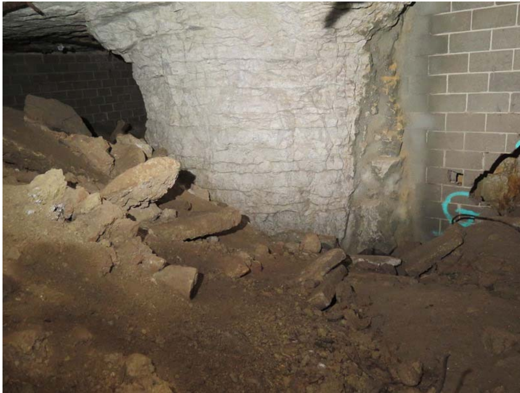
Photo 25: Looking northwest at Pillar 1.
