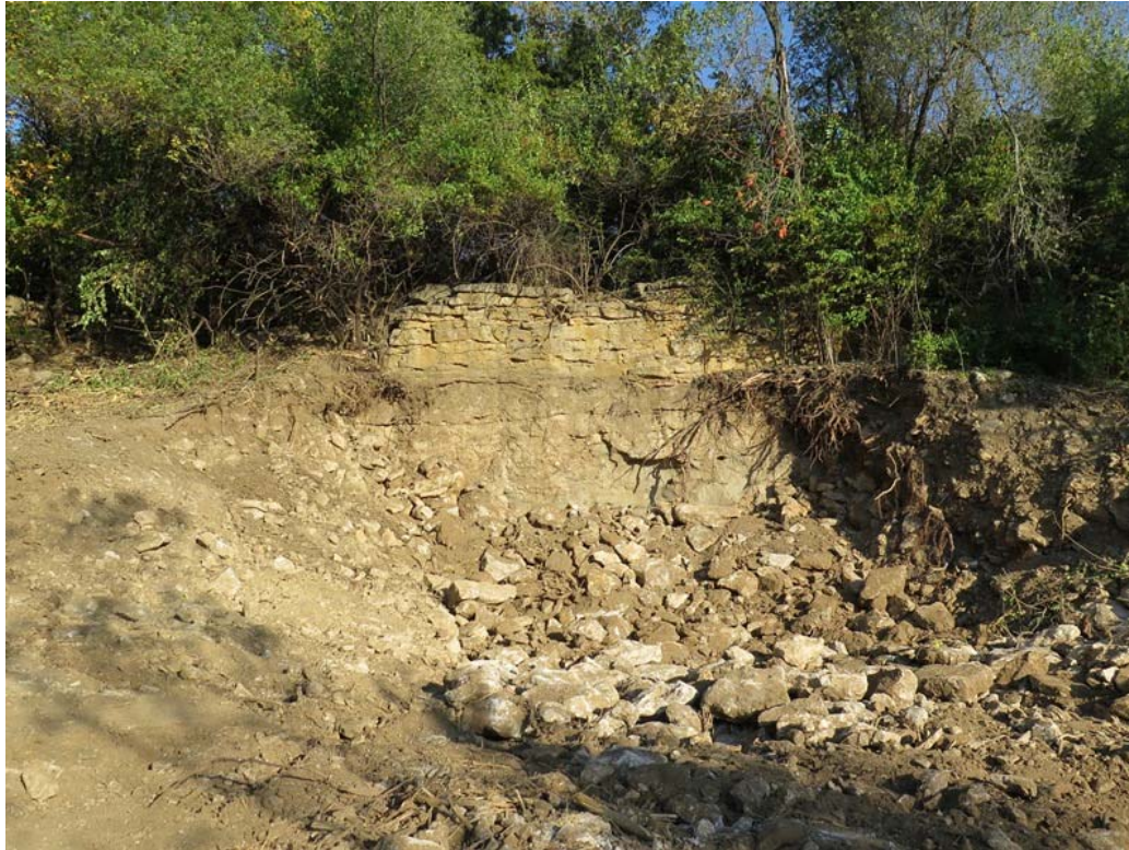
Photo 17: Final backfill of Portal 14, 10/21/15.
