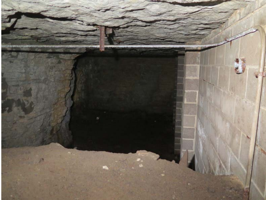
Photo 31: Looking north from Portal 1, Pillar 15 on left, masonry wall on right. Back (north) area is not backfilled.
