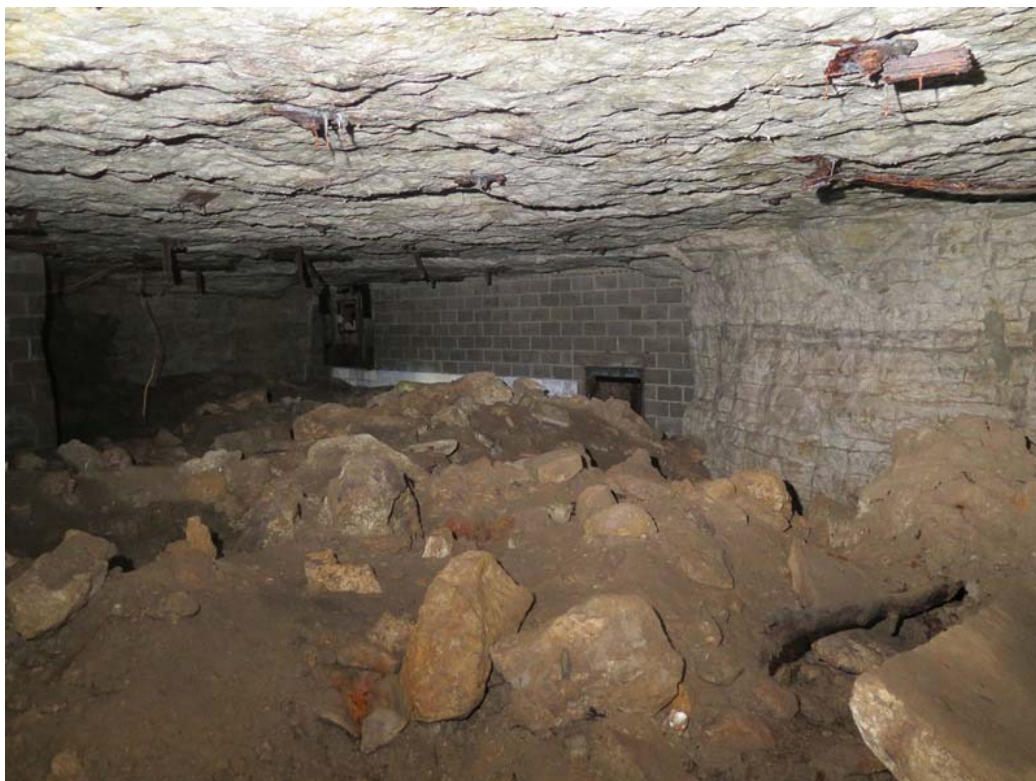
Photo 34: Looking northeast from Portal 3, Pillar 6 on right, Pillar 3 on left. Masonry wall divides supported and developed area from unsupported ground at east of mine that does not appear to have been used for recreational purposes.
