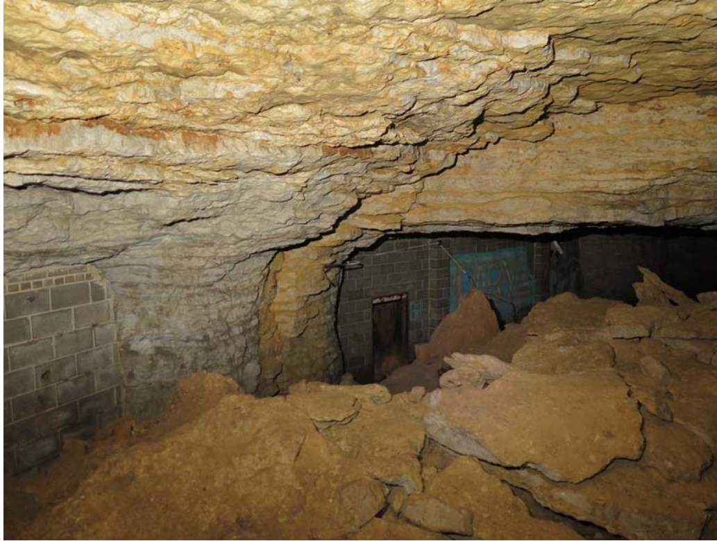
Photo 43: Looking northwest at Pillar 6 and mud seam. Extension of this seam creates the ledge at the back (north) of the dome down on the upper right of the photo.
