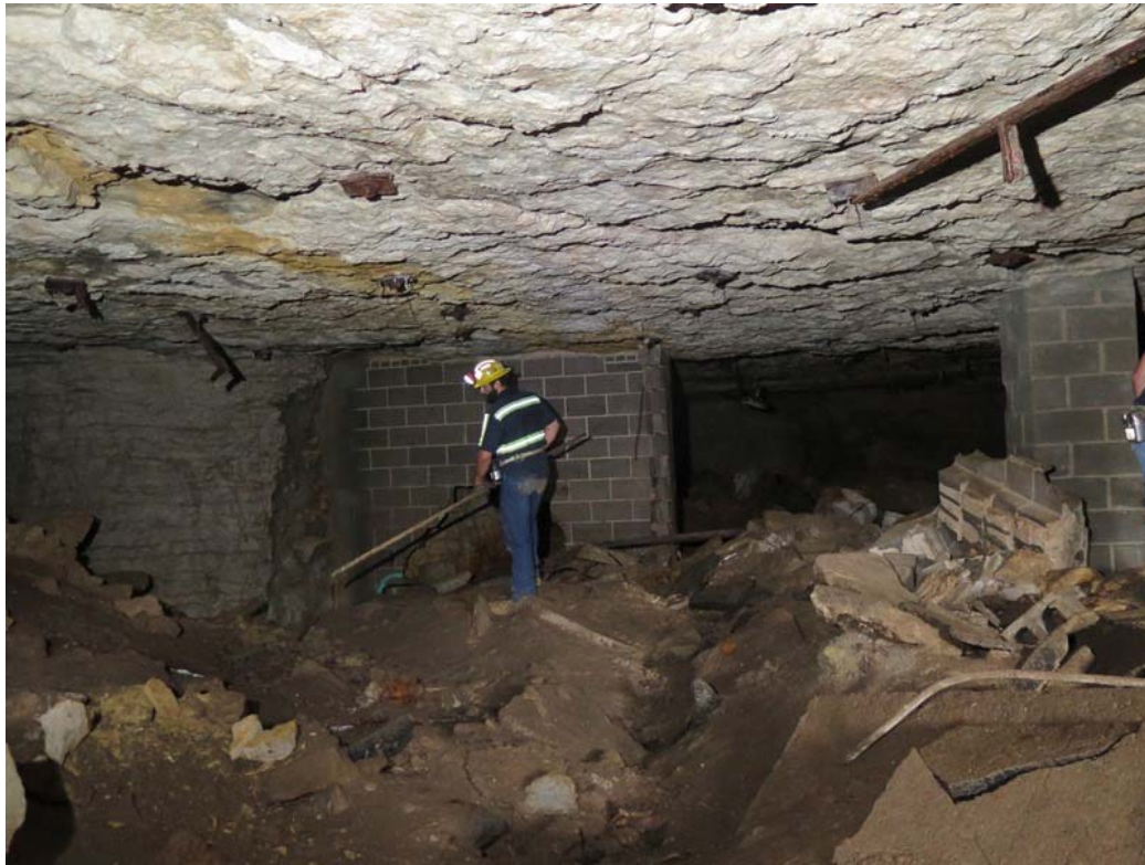
Photo 23: Looking north from Portal 2. Pillar 1 is shown on left, masonry column on right.
