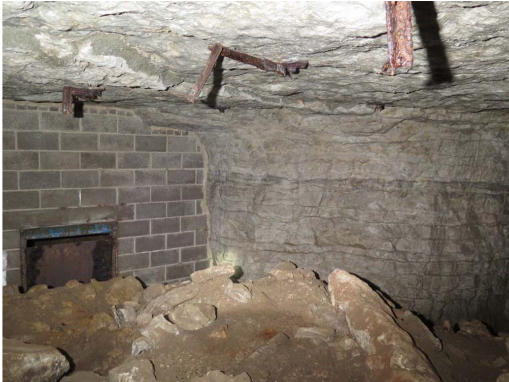
Photo 40: Looking east-southeast at Pillar 6. Door on left is welded shut.
