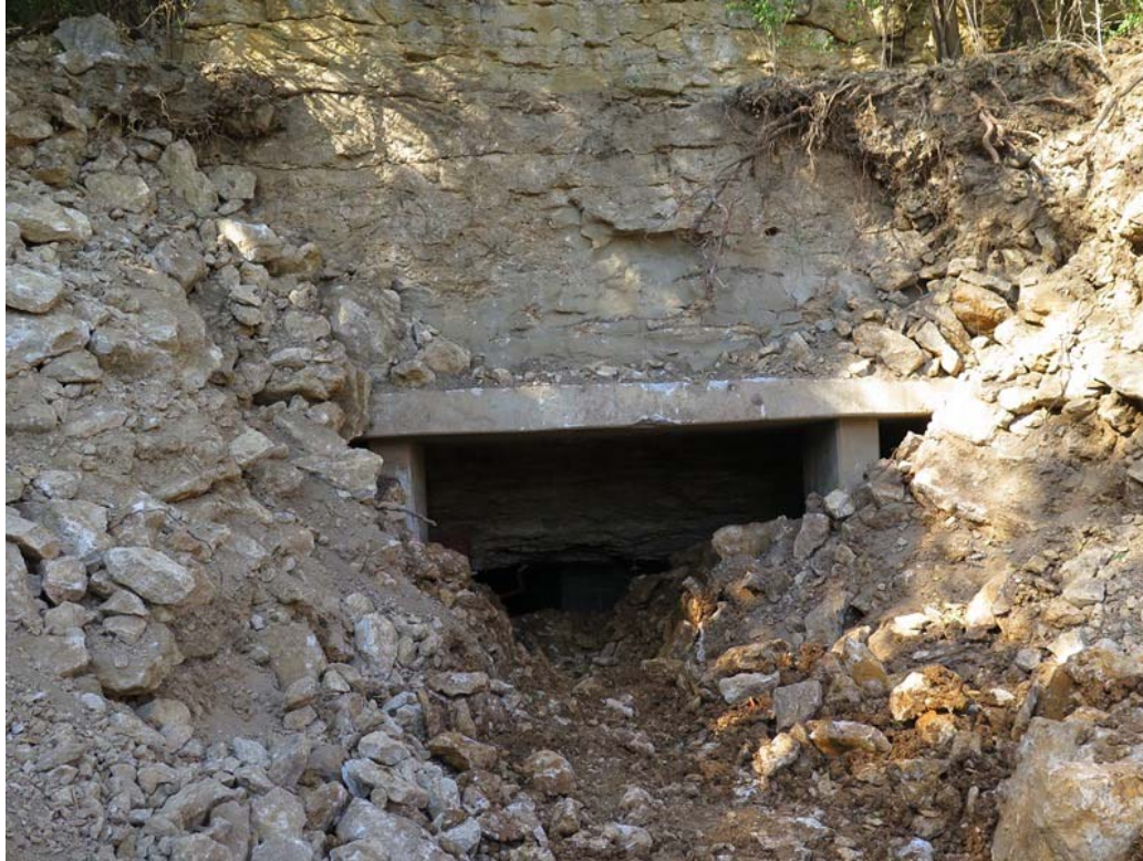
Photo 15: Final Portal 14 excavation.
