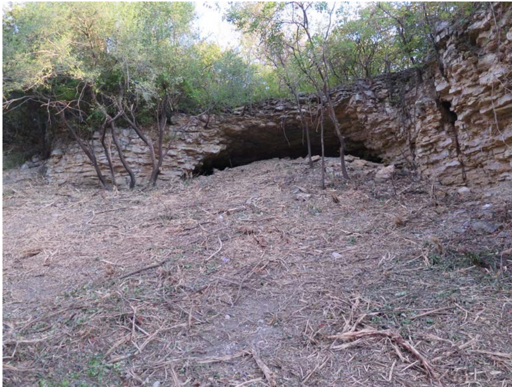
Photo 9: Looking northeast at Portal 6.
