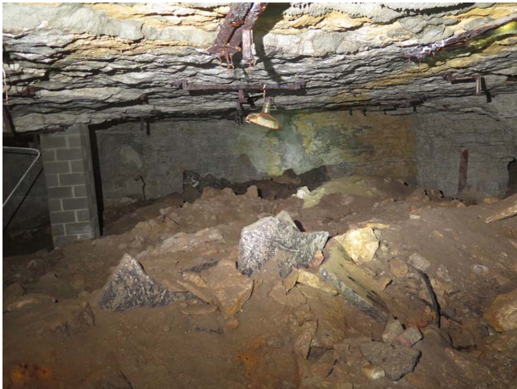
Photo 32: Back (north) room, north of Portal 2. Masonry column on left, Pillar 2 on right.
