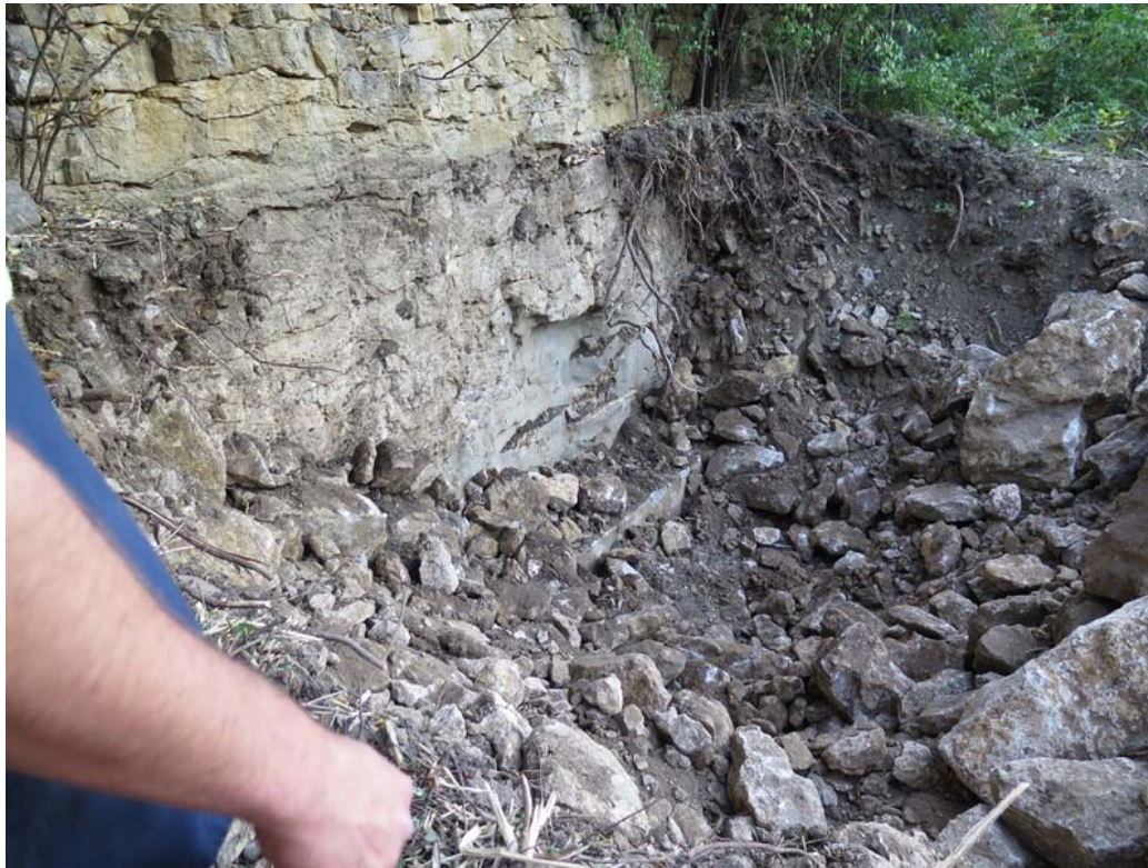
Photo 13: Top of Portal 2 concrete structure excavated. Guniting is visible on the rock face above the concrete.
