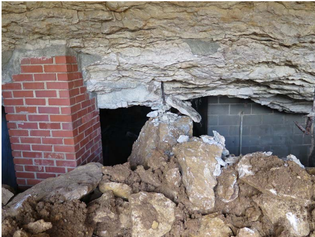
Photo 18: View north into Portal 2. Masonry at right surrounds south and west sides of Pillar 5. Rockbolts in crown exposed at bottom of ledge.
