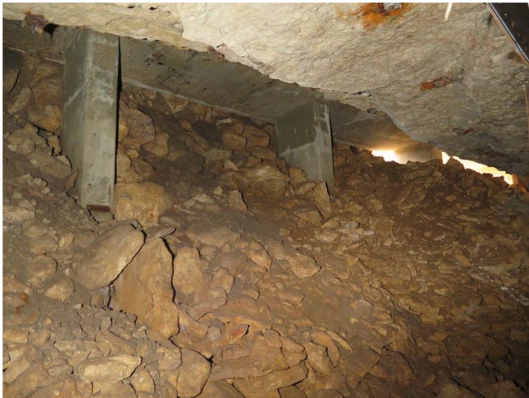
Photo 36: looking southwest from Portal 3 at concrete structure inside Portals 2 and 3. Light visible in upper right is from entry location in Portal 2.
