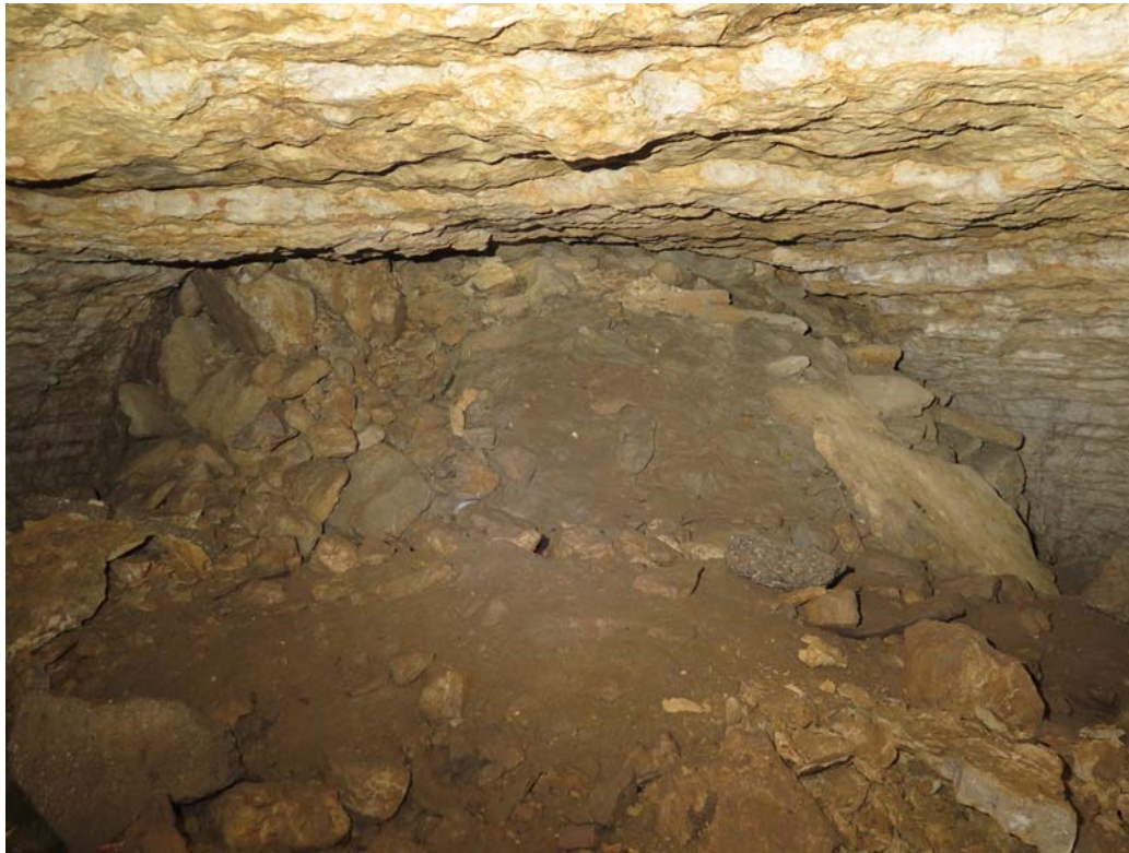
Photo 45: Looking south at Portal 4 backfill. Pillar 10 is shown on the left, Pillar 9 on the right.
