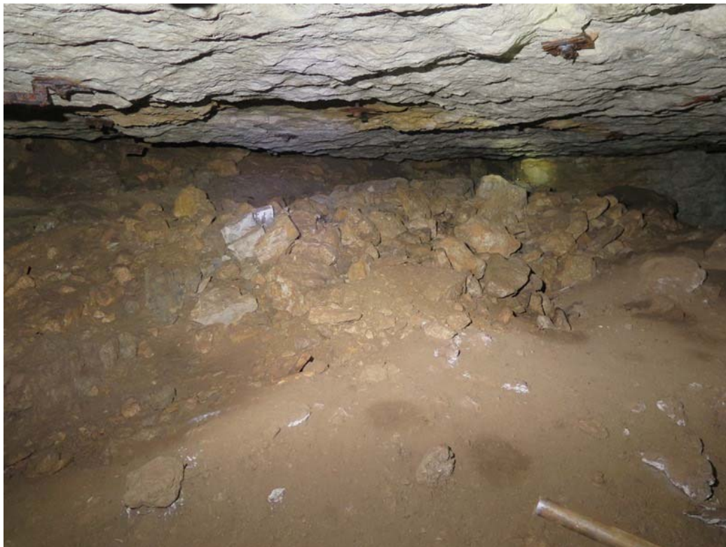
Photo 28: Looking southwest at Portal 1 fill.
