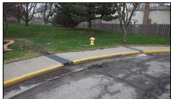
Inlets in southeast corner of parking lot
