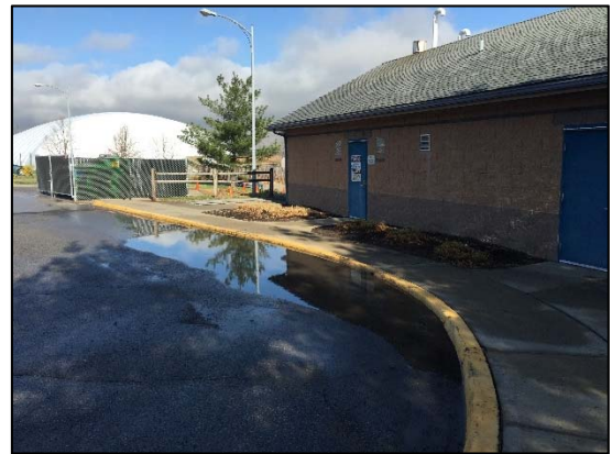
Ponded water at northeast corner of complex (near the pool)
