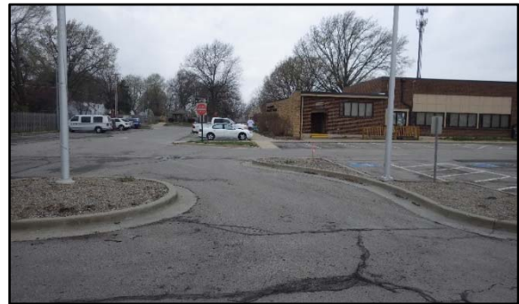
Round-about in southeast area of parking lot
