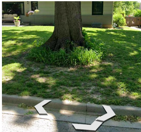
5017: Exposed roots 6.5 LF from B/C, 48" diameter
