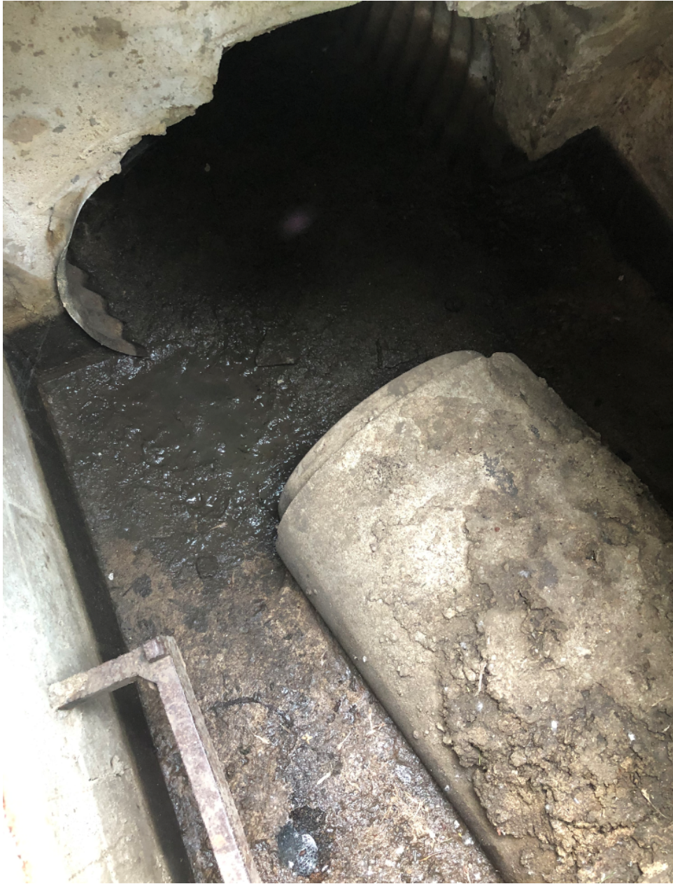
RCP north area inlet. Existing RCP to the north.
