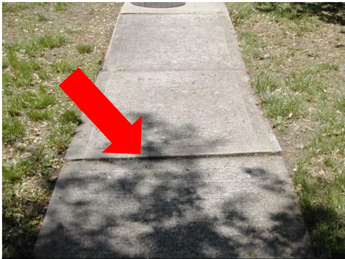
Figure 3L – Faulting ½-1”
