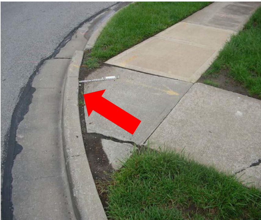
Figure 4H– High Severity Gap
