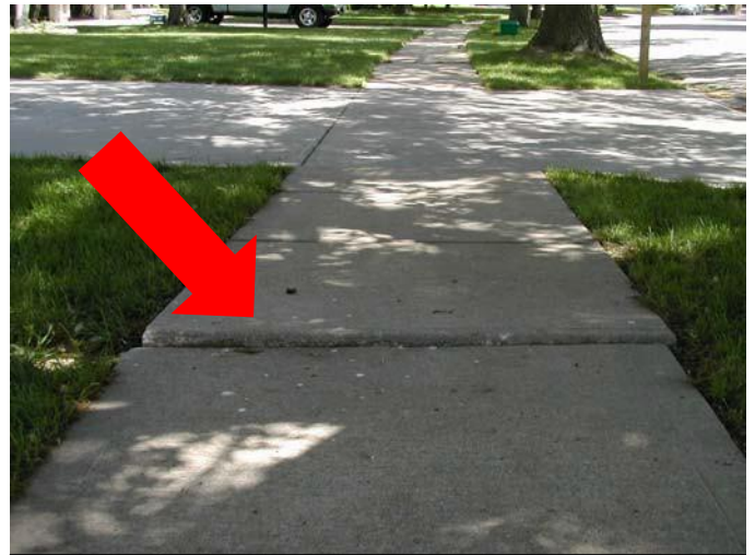
Figure 3M – Faulting 1-2”
