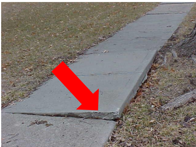
Figure 3H – Faulting >2”
