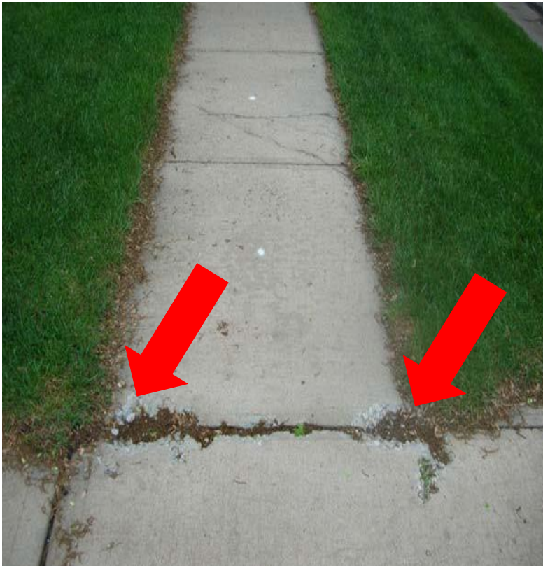
Figure 5L – Low Severity Joint Spalling
