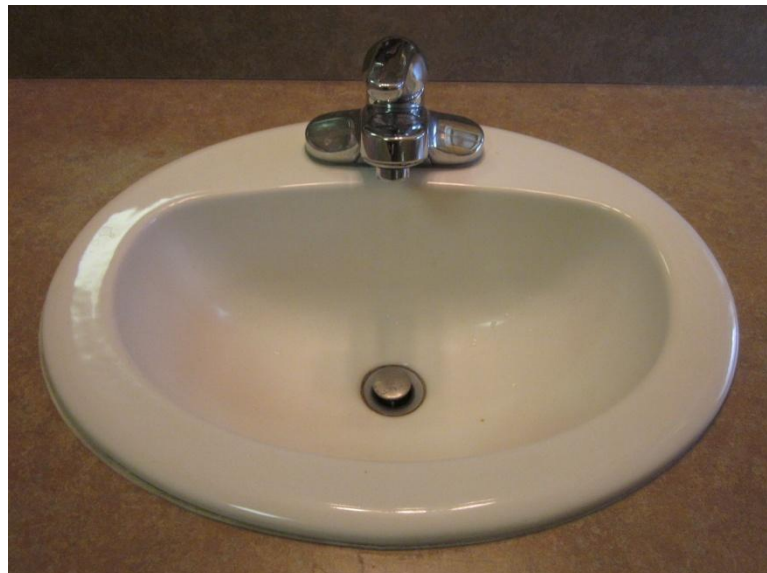
Figure 4.12.B: Typical Lavatory Faucets
