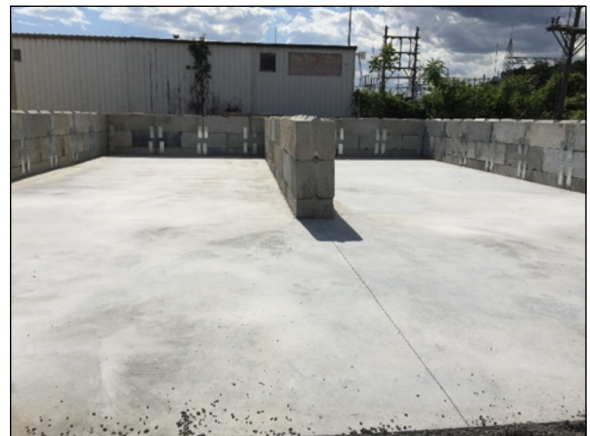
The Concrete Block Walls installed and the Concrete Floor has been poured with separation wall.
