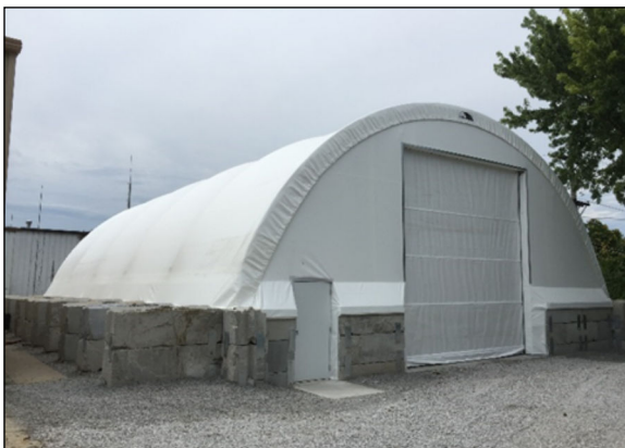
The Concrete Block Walls installed and the Concrete Floor has been poured with separation wall.
