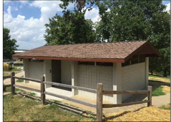
Bathroom was Completely Renovated
