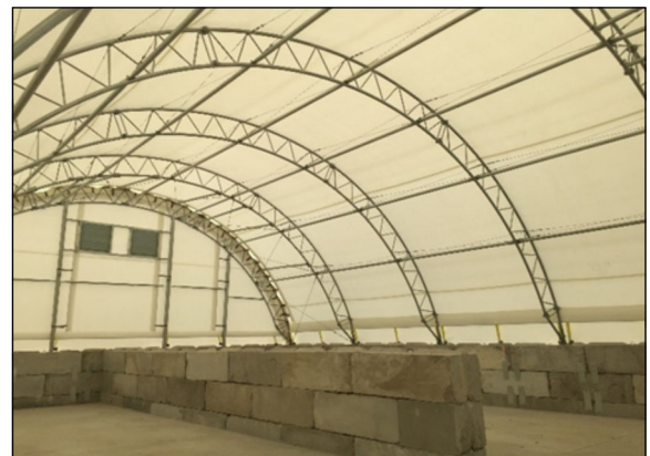
The Concrete Block Walls installed and the Concrete Floor has been poured with separation wall.
