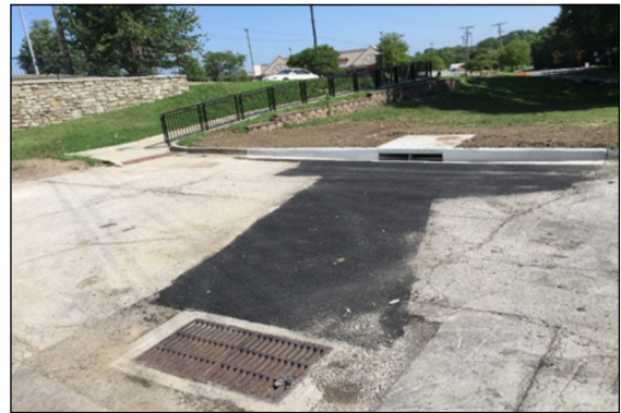
Restoration of Granada Street with new inlet
