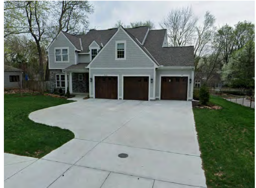
Figure 5.8 - Example of acceptable driveway widths
