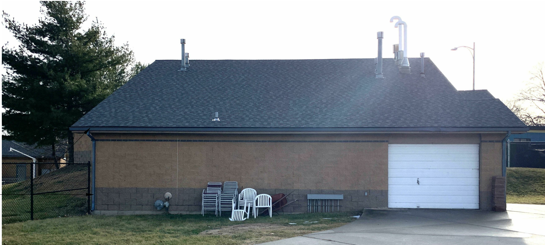
4. PUMP ROOM - NORTH
