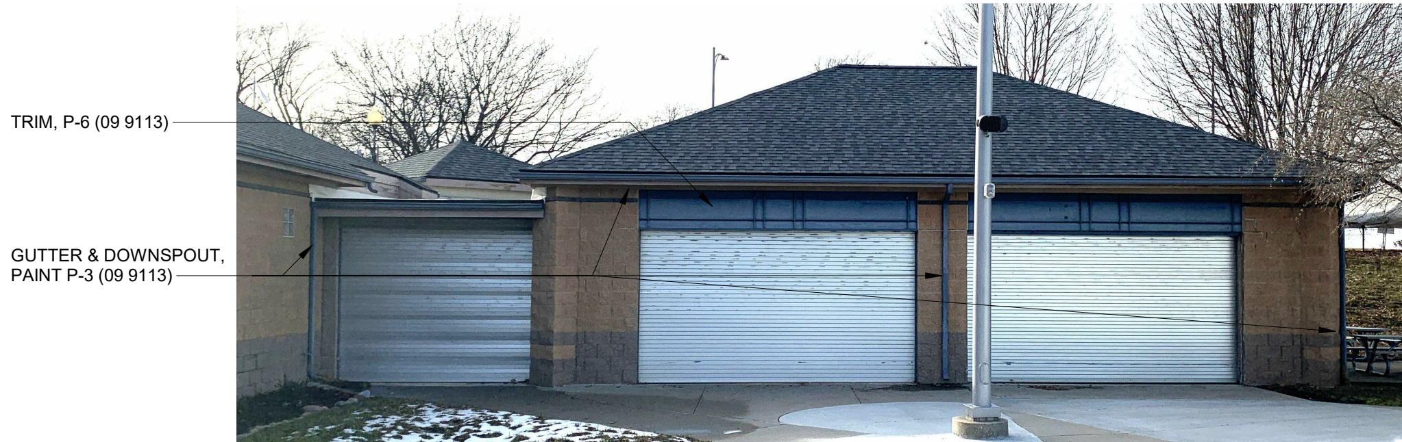
4. BATH HOUSE - EAST 2
