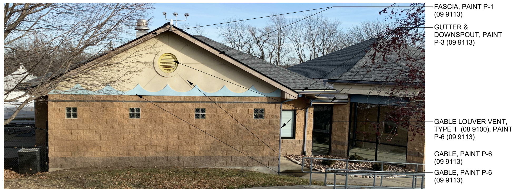
6. BATH HOUSE - WEST 1
