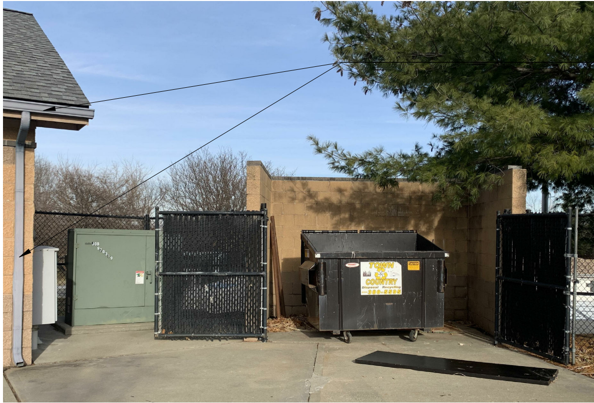
2. PUMP ROOM / TRASH ENCLOSURE - SOUTH
