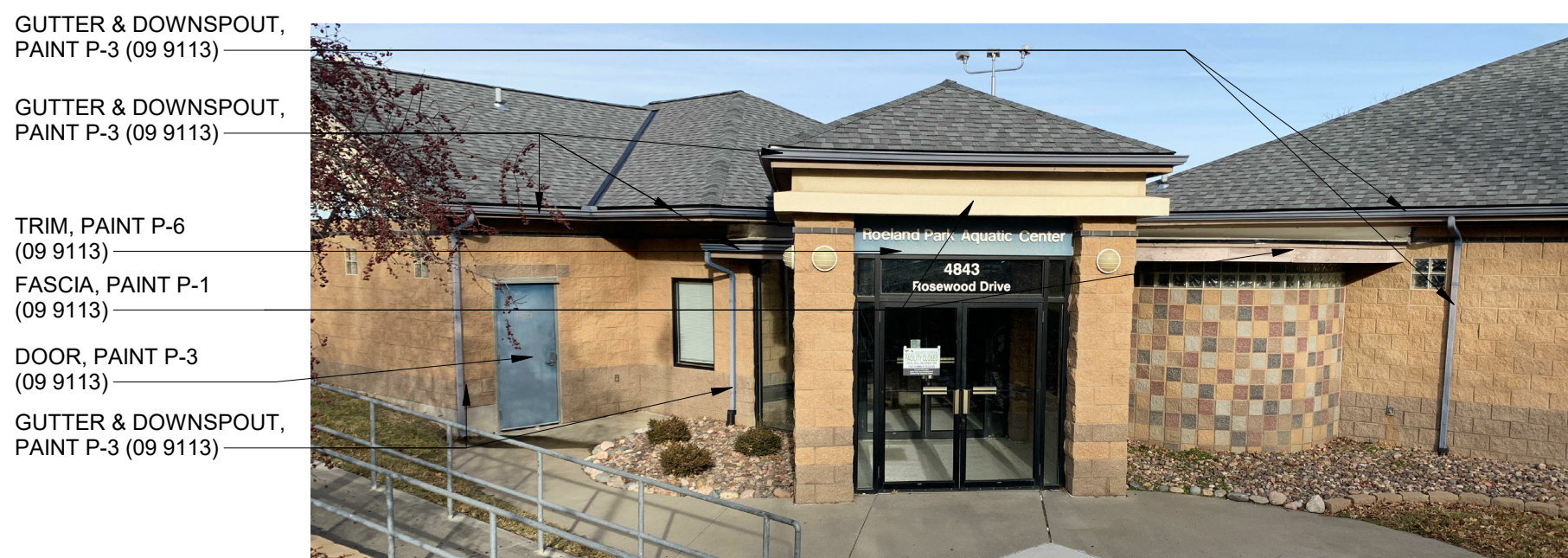
7. BATH HOUSE - SOUTH WEST
