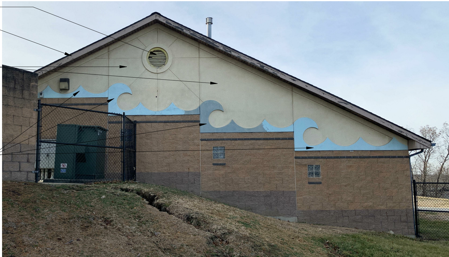
3. PUMP ROOM - EAST
