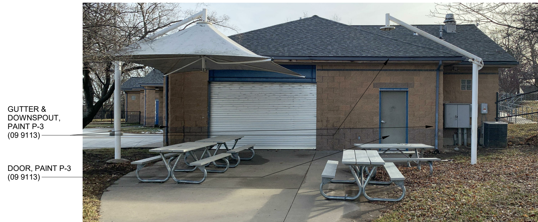
5. BATH HOUSE - NORTH 2
