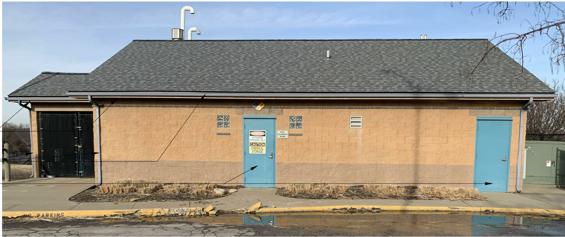
1. PUMP ROOM - SOUTH
