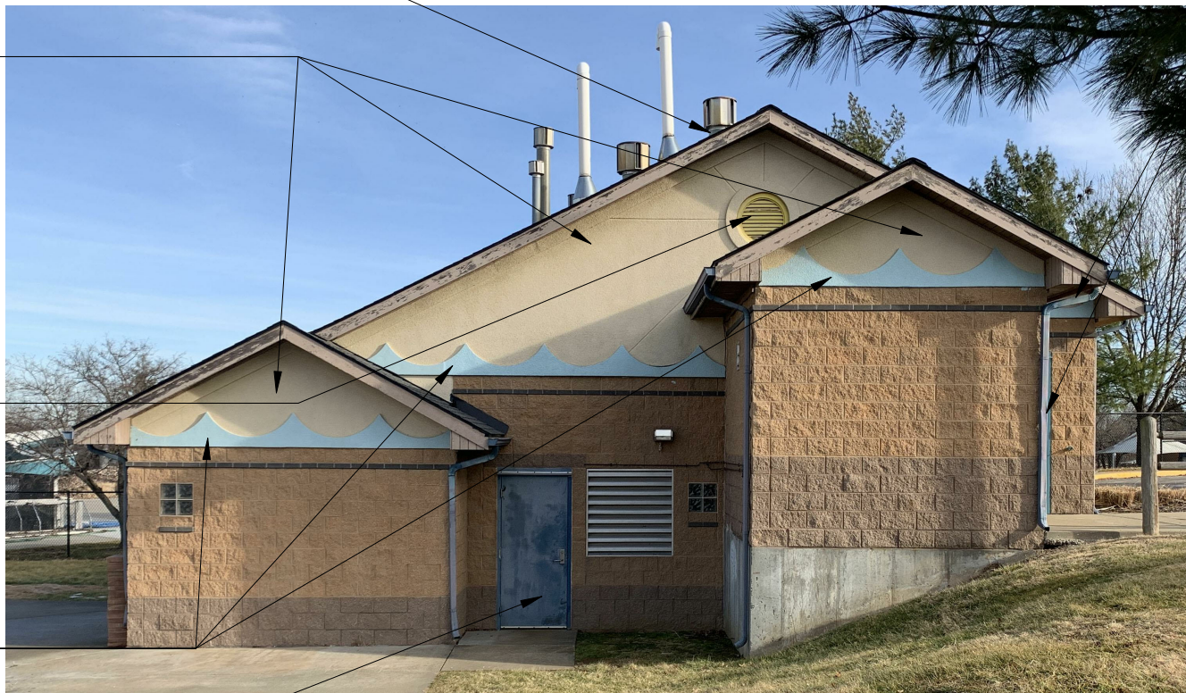
5. PUMP ROOM - WEST
