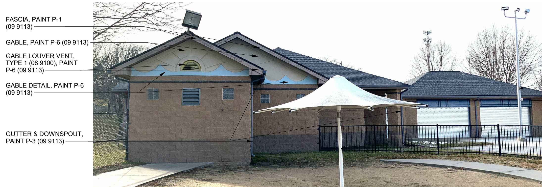
2. BATH HOUSE - EAST 1
