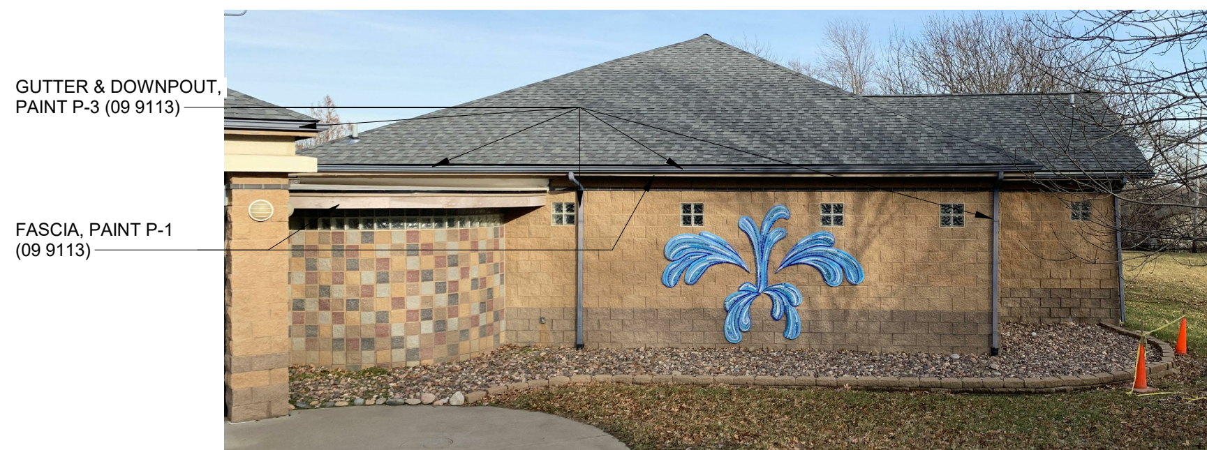
8. BATH HOUSE - WEST 2
