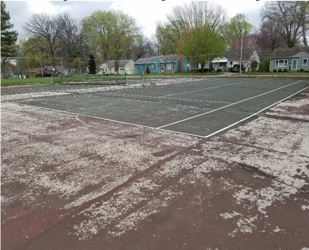
Picture 1- Existing Courts at R Park standing at the NW corner looking SE
