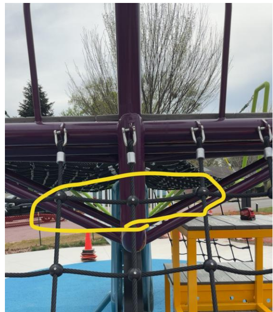
Netting Entrapment – rear of bike
