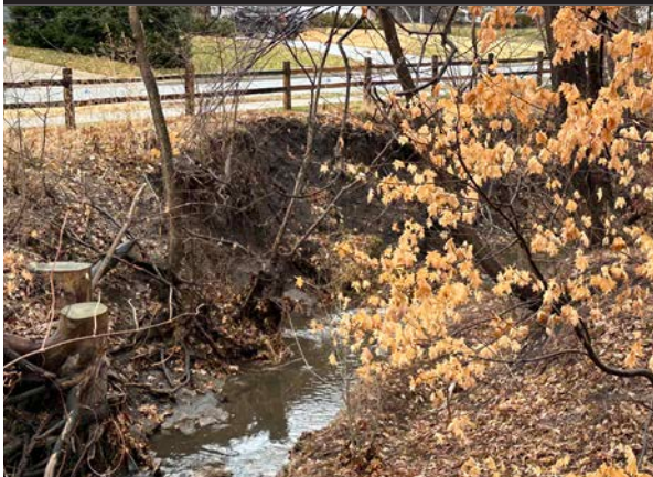
Figure 15. Bank cutting, Reach 2
