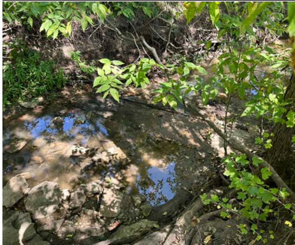
Figure 21. Grade control, Reach 4
