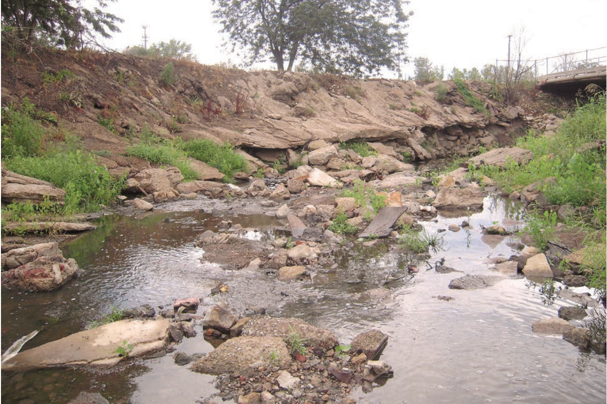
Figure 24. Repaired bank after application of LPSTP
