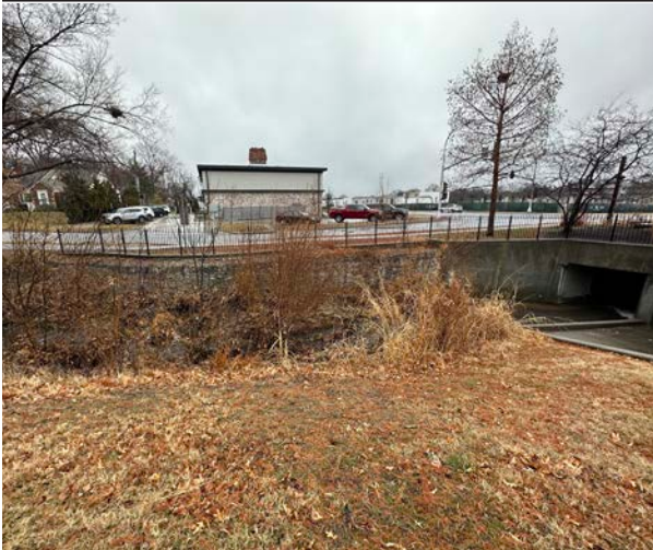
Figure 20. Reach 4 termination at Johnson Drive culvert
