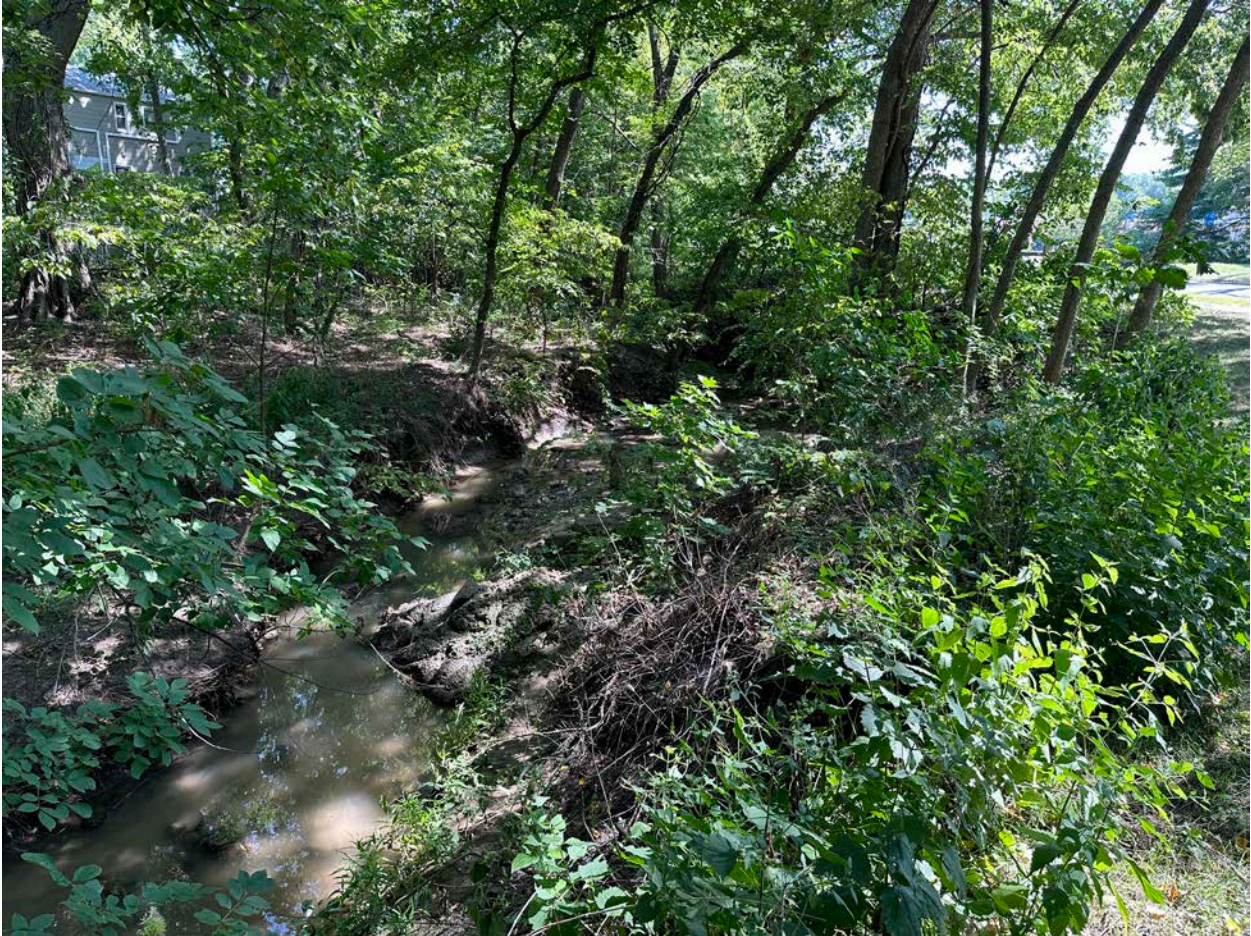
Figure 16. Bank cutting, Reach 3
