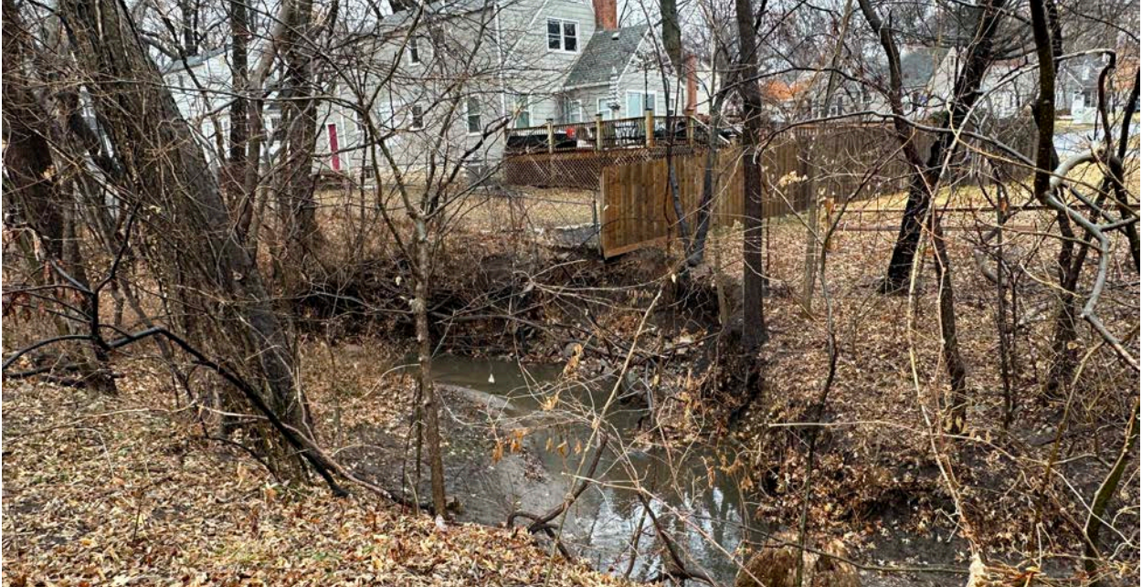
Figure 19. Reach 4 bank cutting behind 5716 Ash Drive
